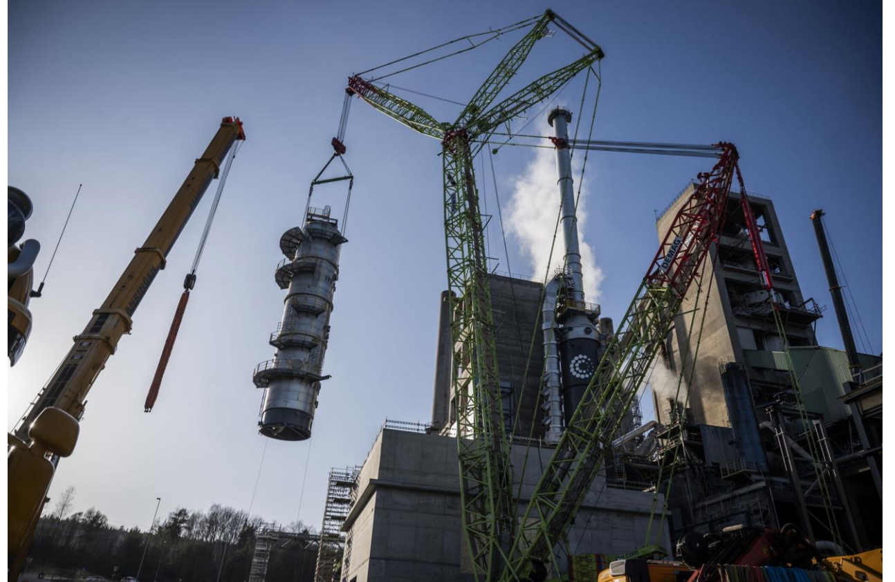
Brevik plant – heavy lifting phase of critical Carbon Capture equipment
