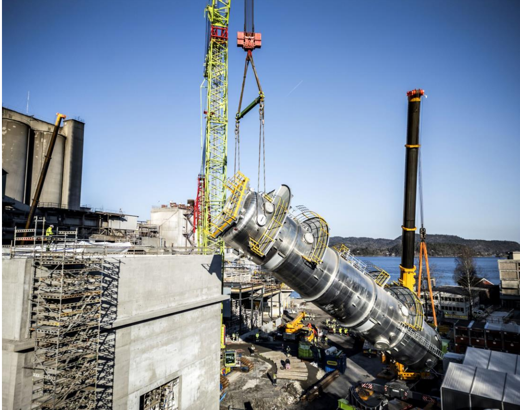
Brevik plant – heavy lifting phase of critical Carbon Capture equipment
